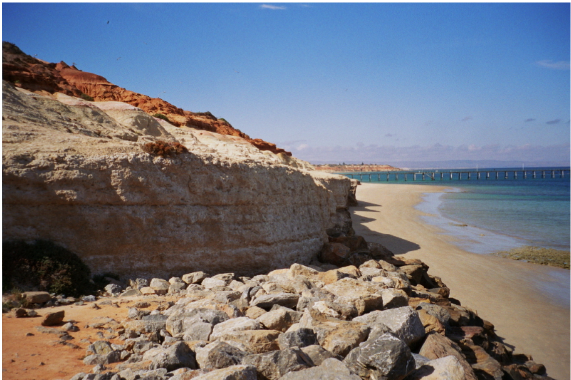
Plate 8 Southern end of rock armoured slope protecting existing base trail at Witton Bluff, and commencement of limestone base platform beyond, that is present over northern half of project site
