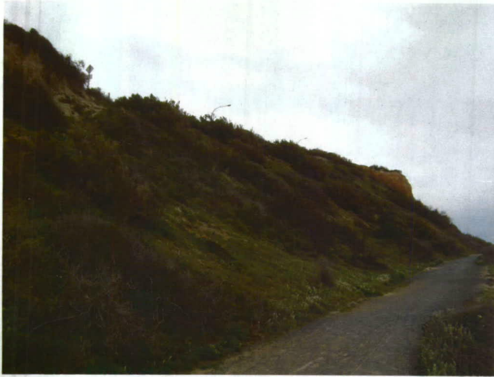
Plate 12: General view from walkway looking south towards a cliff zone of typical 1V:1H (45°) vegetated slopes.
