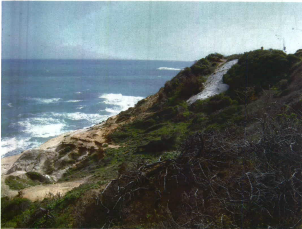
Plate 31: View looking north across an old backfilled backscar and white hydromulch and jute covered remediated slope. Upper slope is well vegetated.
