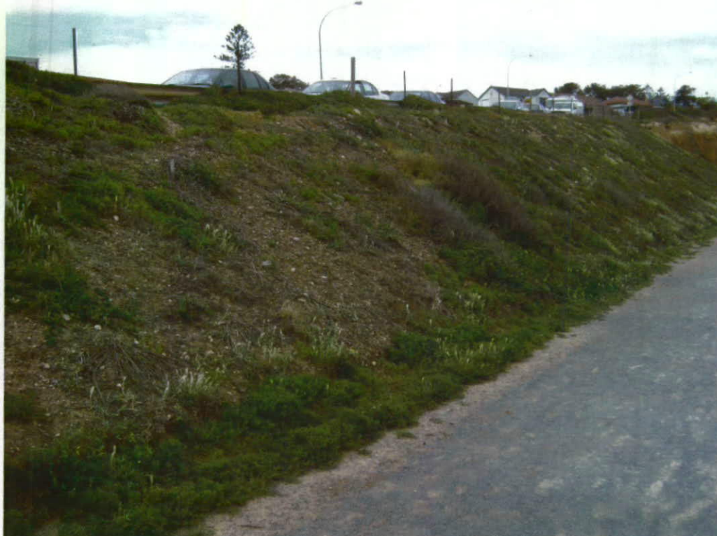
Plate 3: General view of the slope, from the walking path, looking to south at a zone of 1V:1H (45°) slopes. Patchy vegetation with jute and enviromat covering the slope.
