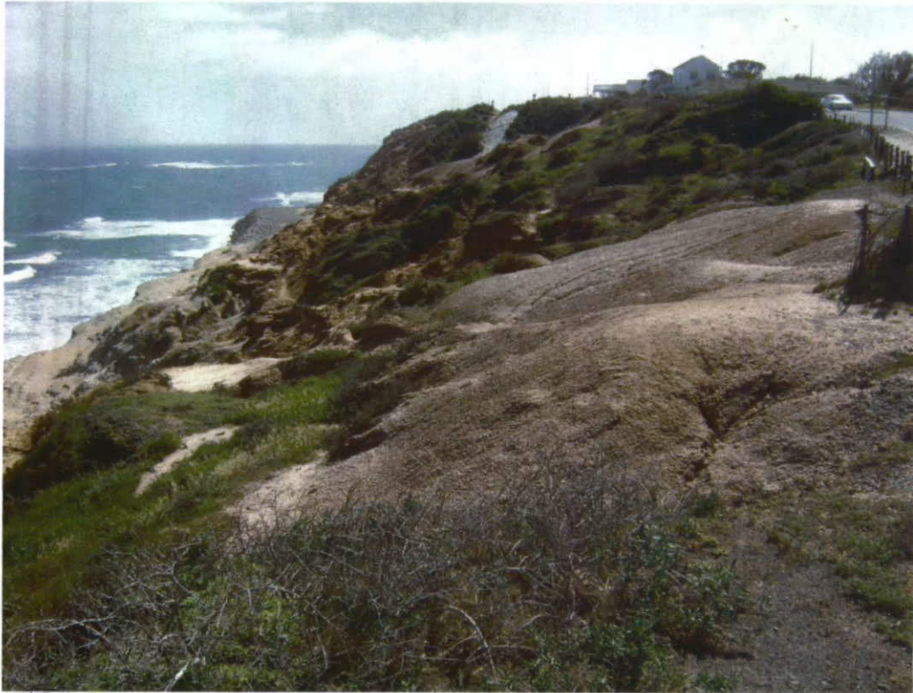
Plate 43: General view north at slopes 30 m high, 1V:1.7H (30° inclination), crest at edge of road.
