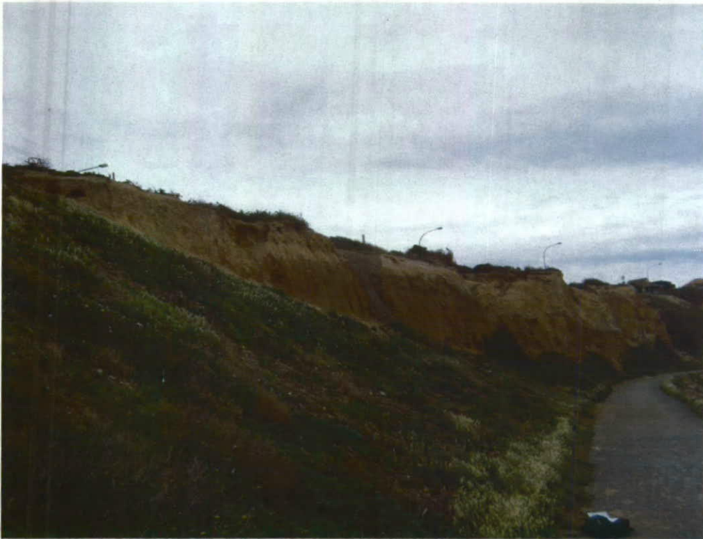
Plate 4: General view from the walking path, looking to south, at a zone with slopes 1V:1H (45°) to 2V:1H (60°). Zone has a danger sign 'Falling Rock' in the middle of the area adjacent to the walkway.
