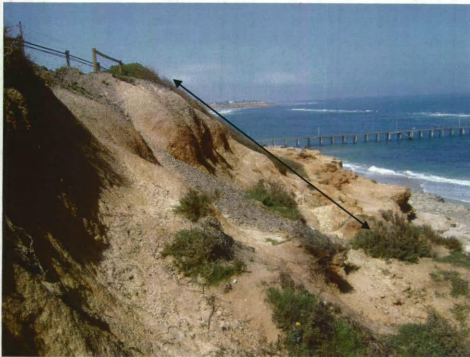
Plate 44: General view south highlighting the proximity of the road to the crest of the cliff slope immediately above the coastal site of active cave formation and recent rock falls. Slope 30 m high, 1V:0.7H (55° inclination).
