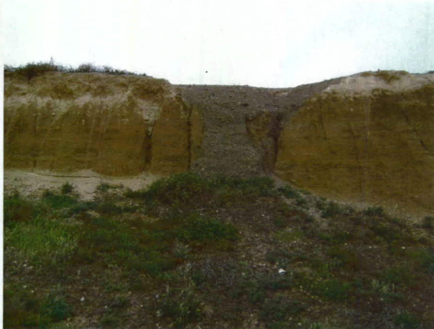
Plate 5: Localised crest erosion remediated in the past with a thin covering of concrete. Concrete partially intact due to erosion. Ongoing minor crest erosion.
