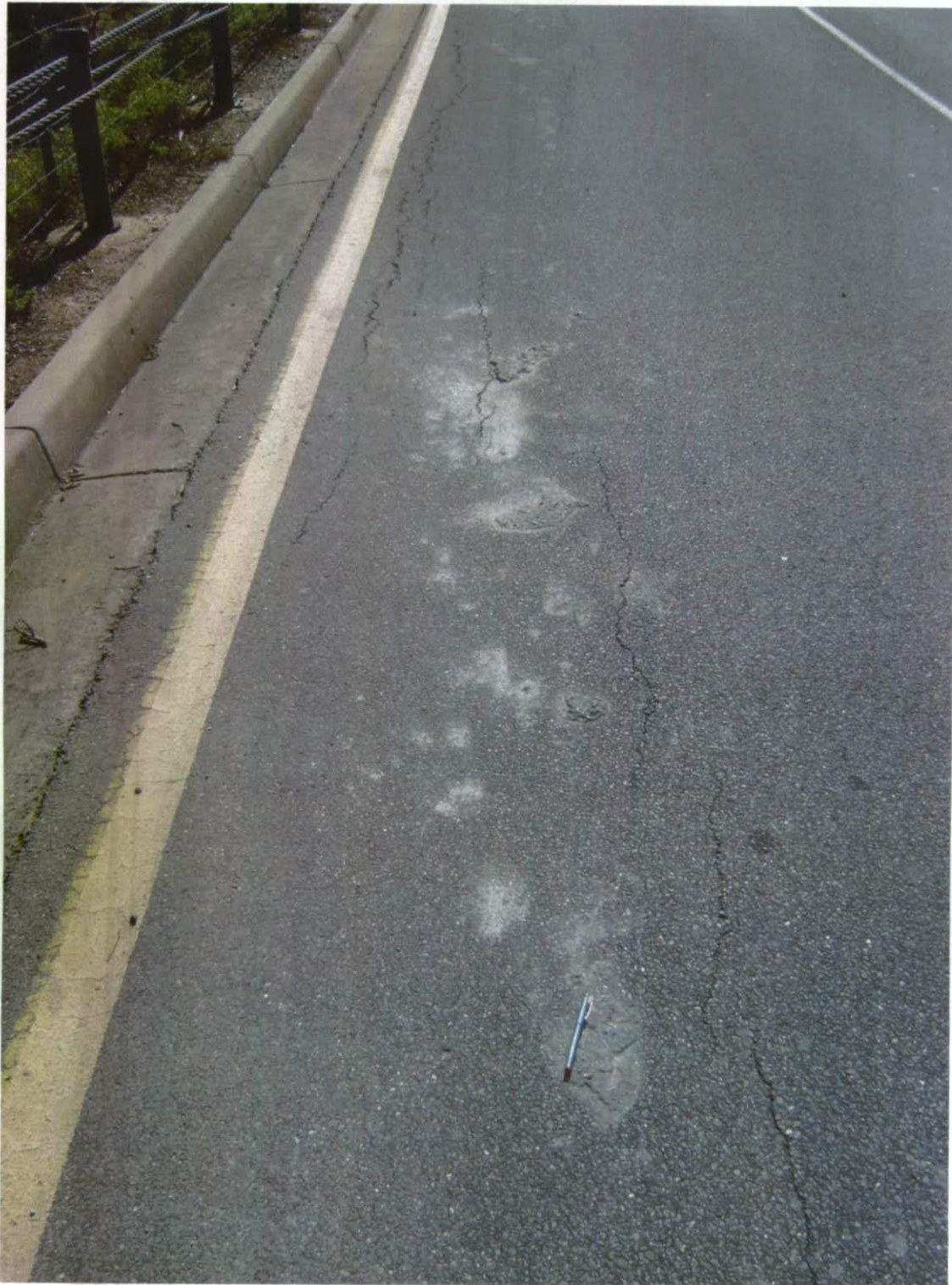
Plate 16: Hairline longitudinal tension cracks on the road
