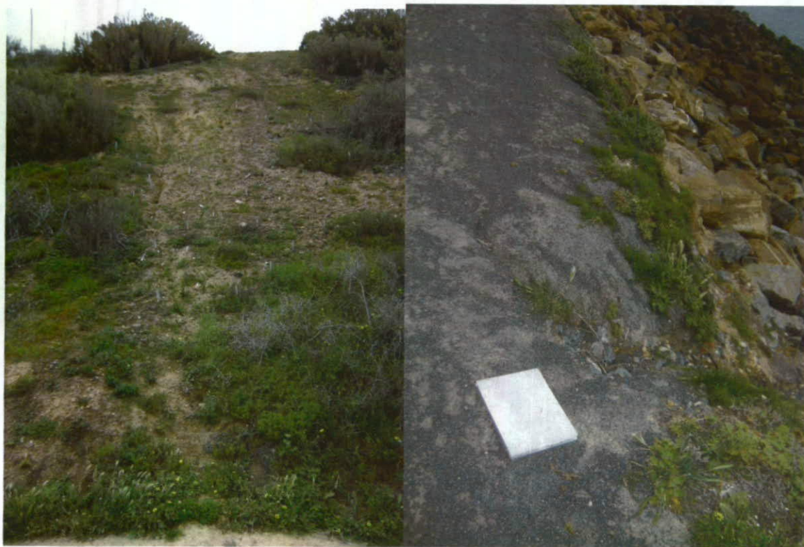
Plate 13: Water erosion has led to rill erosion of sandy soils (left photo) and of the edge of walkways (right photo).
