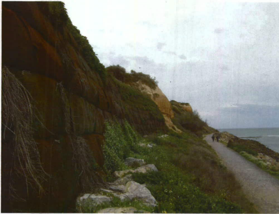
Plate 8: View looking south, at the base of the reinforced earth retaining wall. Wall has limited vegetation and some areas where the jute is torn.
