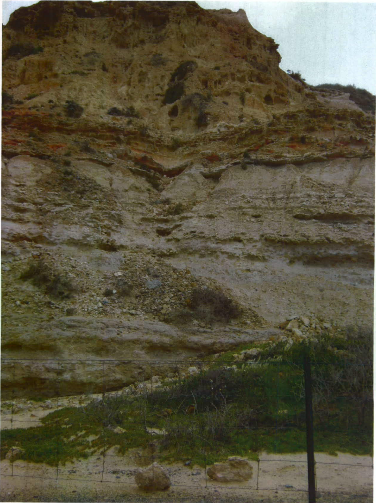
Plate 23: View looking east (towards Benny Avenue) at a typical slope covered with small rocks. Note the dominance of voids and undercut sections in all sections of the slope.
