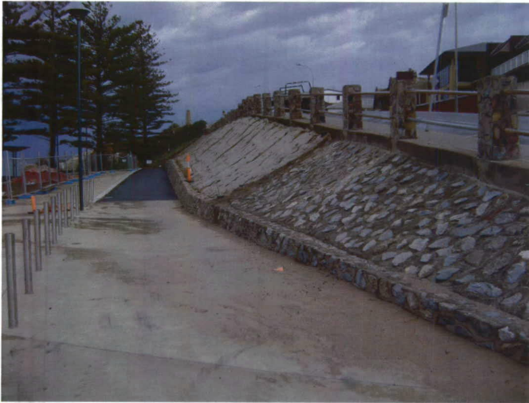
Plate 50: View looking north along Zone O and Zone N. To the left of the orange beacon, work was in progress placing the erosion protection matting and planting seedling in the slope.
