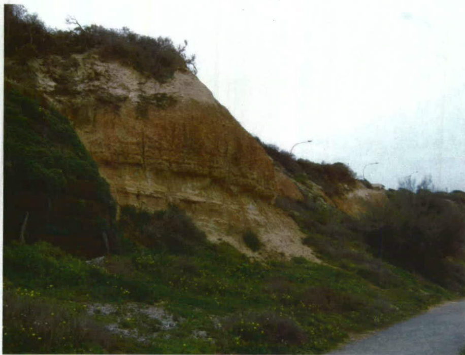
Plate 9: Southern end of retaining wall, cliff erosion is uneven, leading to shallow slopes at crest and undercut sections in the lower portion of the cliff face. No danger signs displayed.
