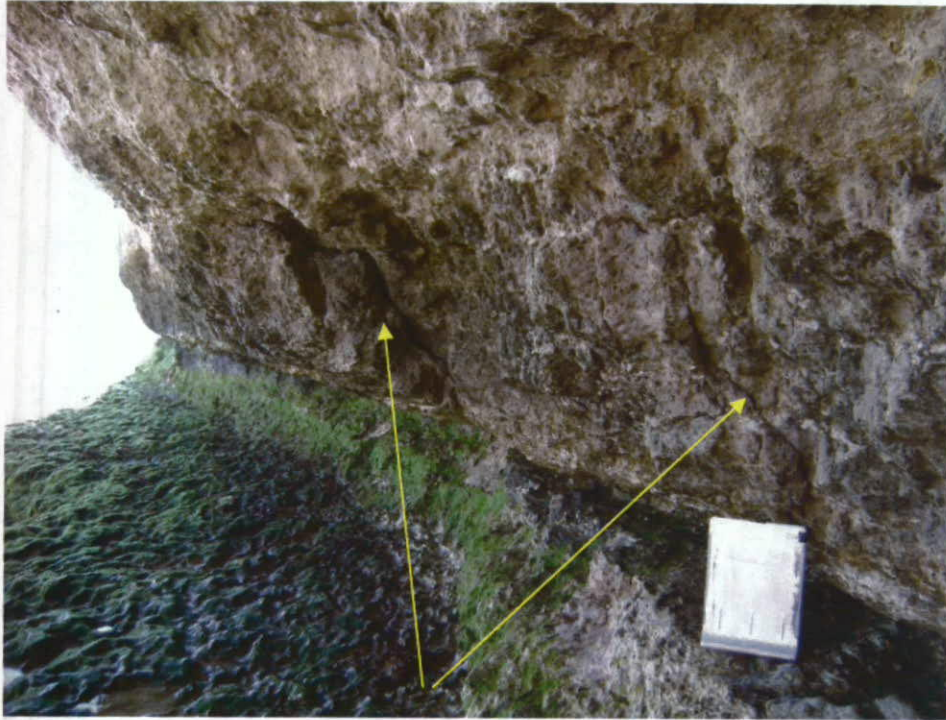
Plate 40: View of shallow seated scalloping fracturing of the rock, above the moss covered tidal influenced wave cut platform. Cracks will lead to failure of the rock in the short term.
