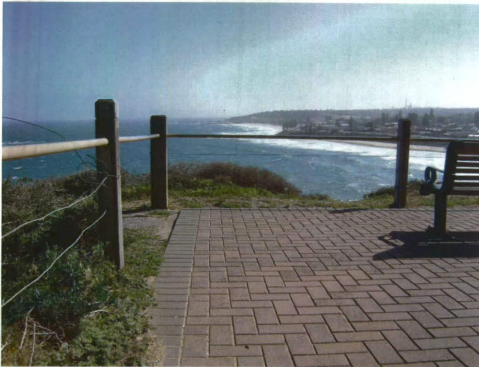
Plate 21: View looking north at broken wires in the lower section of the fence at Witton Bluff Look Out.
