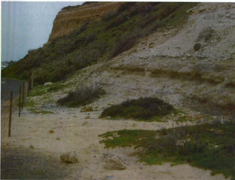
Plate 22: View looking north at the base of the slope. Note the fence and the small 120 x 200 x 300 mm low strength rocks on the walkway.
