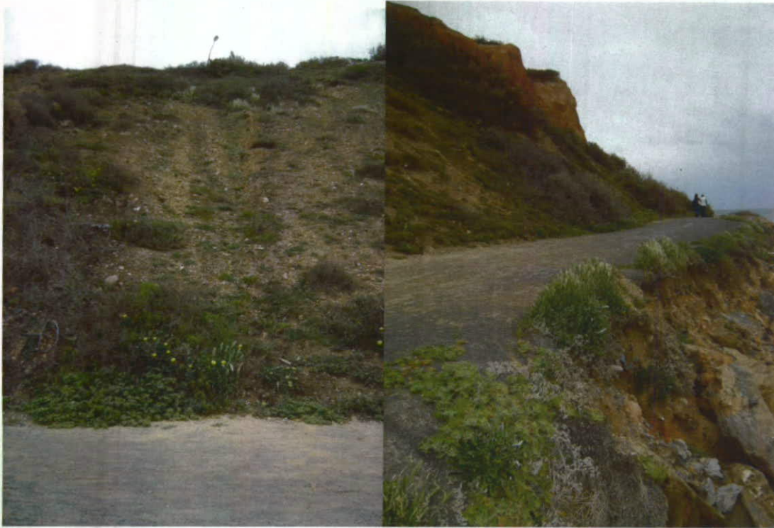
Plate 14: Water erosion has led to rill erosion of sandy slopes (left photo) and of the edge of walkways (right photo).
