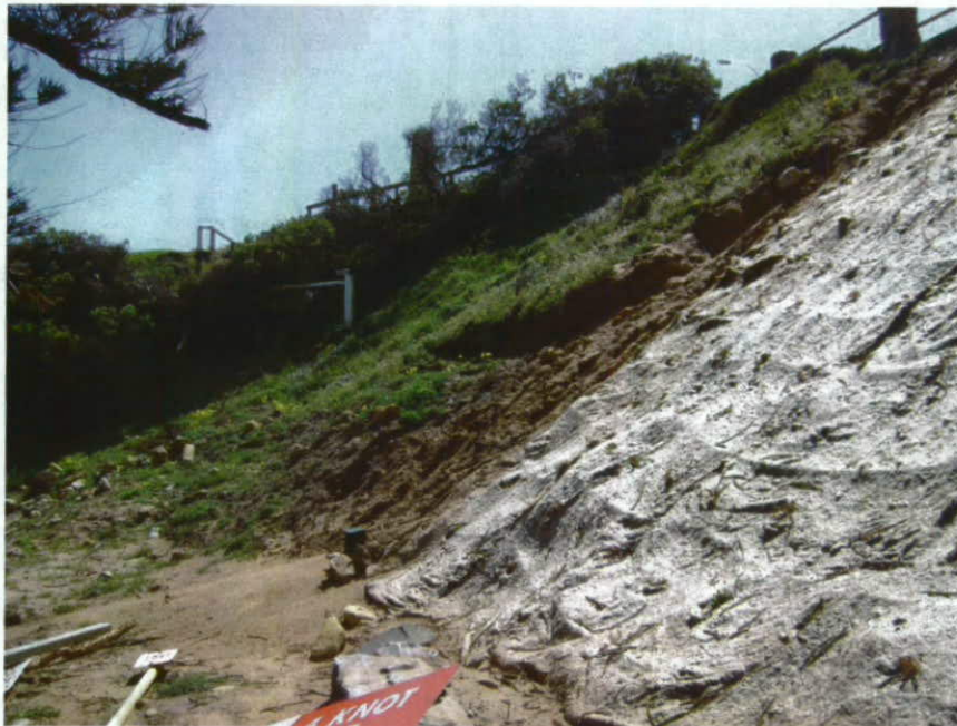
Plate 49: View looking north at Zone N where the remediated slope abuts a stone and cement rock armour of the slope. This armouring has been recently disturbed and through time will expose soils to erosion.
