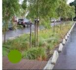
Swales, detention basins and WSUD integration to car parks are essential techniques for the treatment of stormwater across ASP. The adjacent stormwater plan indicates locations of stormwater treatment types and the above images illustrate what these swales and basin may look like within ASP.
